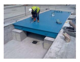
For surface mounting a simple flat concrete slab is required with ramps to 400mm.
